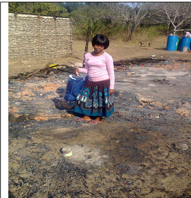
Figure 5: Ms.Ndabandaba (Completely damaged house)
