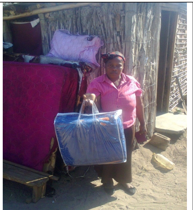
Figure 6: Ms.Ndlovu (Partially damaged house)
